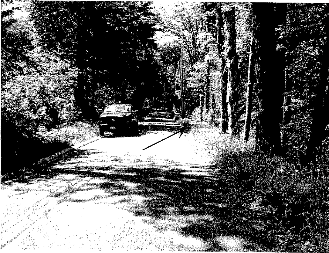
263 Long Pond Road Looking South
